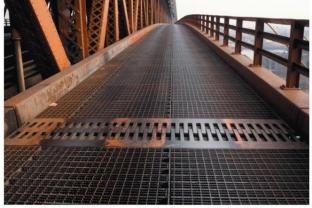
**Expanding spans:** A long steel bridge will slightly increase in length on a hot day and decrease on a cold day. Thermal expansion joints let the bridge's length change without causing the roadway to buckle.
